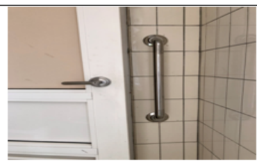
廁所設置扶手後
